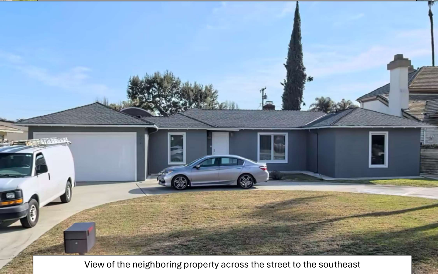
View of the neighboring property directly across the street
